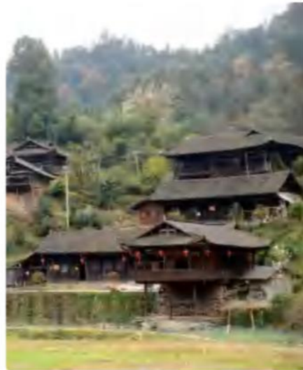
土家吊脚楼 Tujia Stilted Houses
